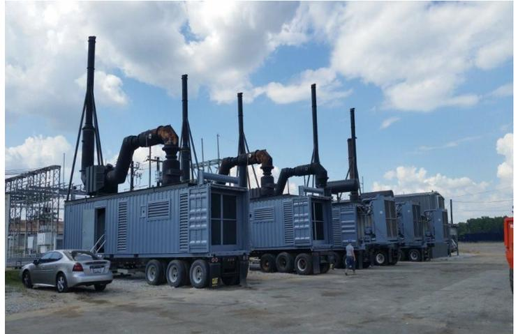
**Colton Power – Drews Power Plant and Century Power Plant – California, USA** Walters Power International and investors acquired two 40MW power plants in southern California. These two plants are powered by eight GE GT10 gas turbine generators with extensive emission control packages. These plants were operated for several years in the California Resource Adequacy market. They were sold to an investor group in early 2016.
